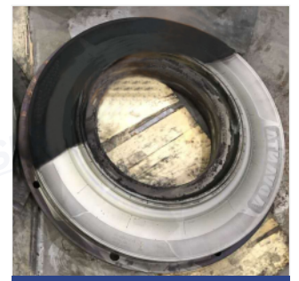
● Remove coating on flange surface
